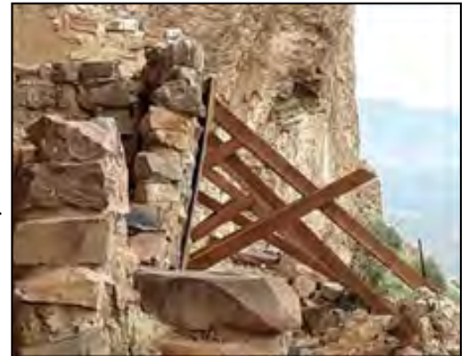
Wooden Braces Holding Up Wall at Tonto National Monument
