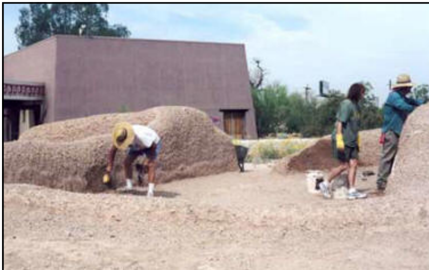
The "Pueblo Grande Mudslingers" began as a Southwest Archaeological Team (SWAT) project in the 1990s. Here the group works on the stabilization of the Pueblo Grande platform mound, Pueblo Grande Museum and Cultural Park, Phoenix.
