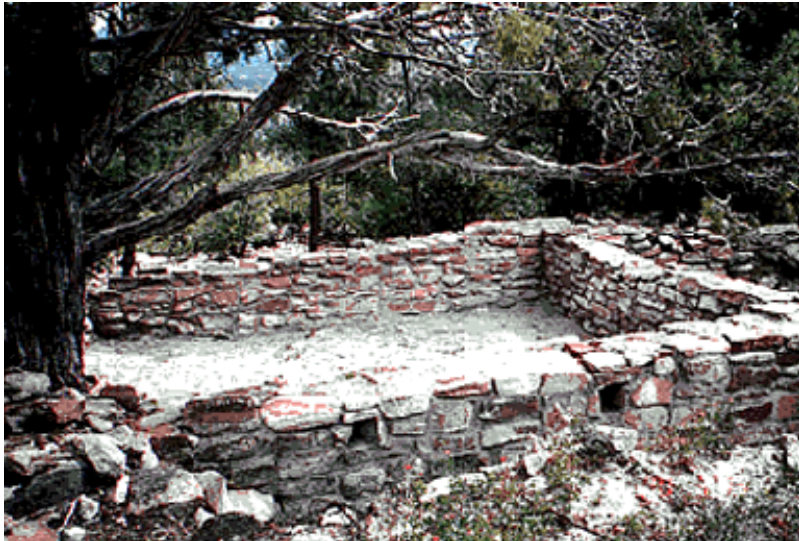
Completed Room 8 west wall. Note 3 vent holes
