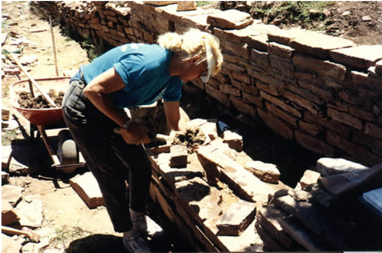
Marie reconstructing a course on the east wall of the entry way into Room 15. The wall behind is the 1990 stabilization project done by J. Britton and J. Bashaw.
